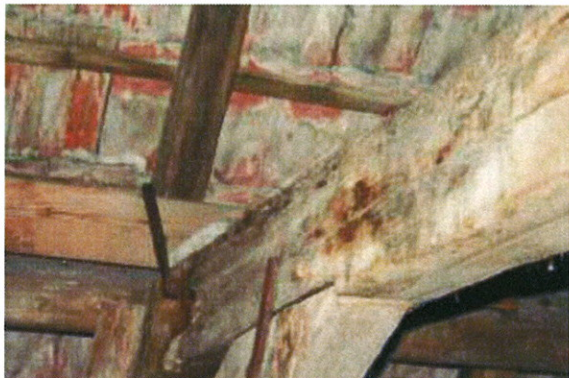
Obr. S51 – Detail ležatej stolice
